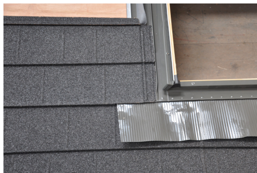
Fakro Tile Flashing installed with Guardian Roof Tile
