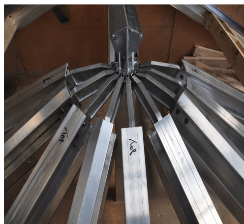
Typical Spider assembly using pins and locking nuts provided
