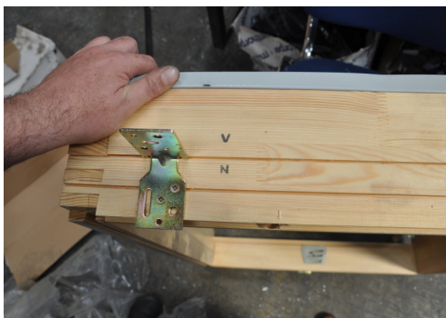
Fakro Window to be fitted to the V Notch
