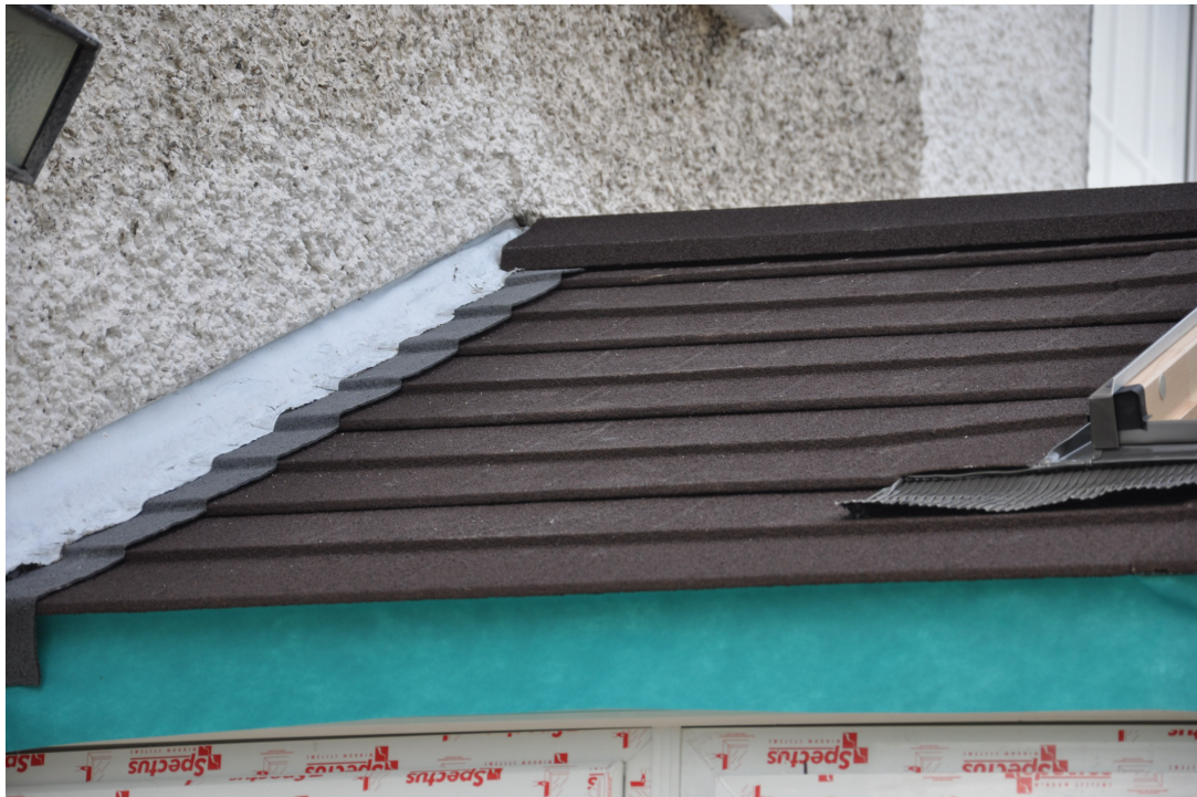
Fakro Tile Flashing installed with Guardian Roof Tile
